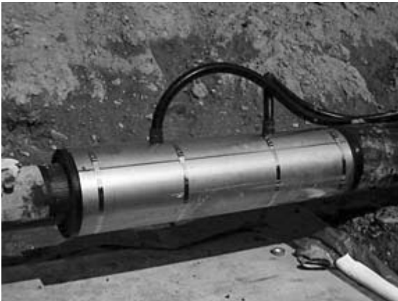
28.2 An FSM-IT installation with protective cover.
