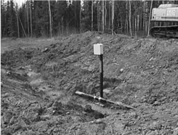
28.3 An FSM-IT installation before earth filling.
